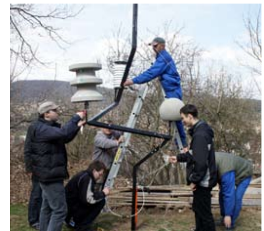
Installation of the measuring system assisting location-specific planning
